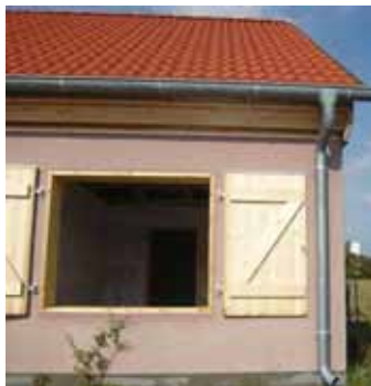
Typical building in the target area
